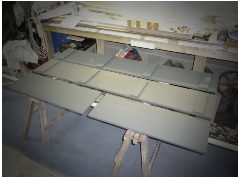
Right – Back to the carpentry, the sides and ends receive two coats of Dark Grey undercoat. It's now early February 2011.
