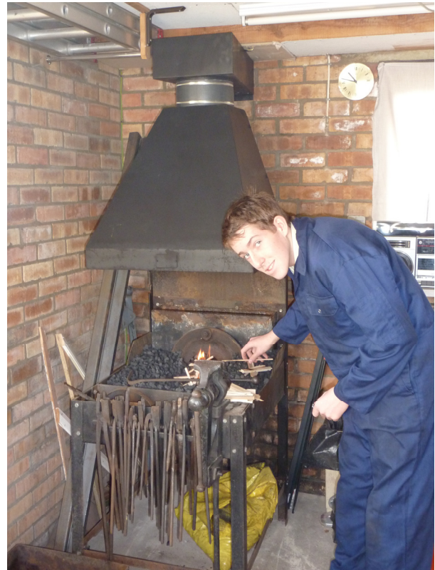
Right - The forge had been retrieved from the trailer and installed in the workshop early in October. The 11" diameter spigot on the cowl required a flue transition box to connect it to the 115 2 chimney. The chimney had been incorporated into the workshop when built, back in 1996, in anticipation of some form of combustion chamber. A manual damper is incorporated to keep the birds and draughts out when the forge is not in use. Alistair is caught about to light the kindling under the coke nuts for the first time, while his dad contemplates the probable results of same.
